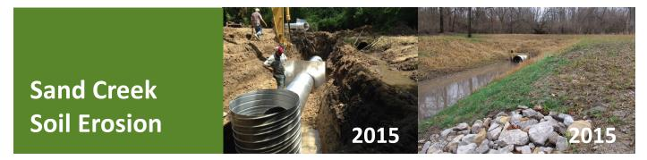
This drainage and erosion control project along a trail at Sand Creek Conservation Area was completed in 2015. It improves water quality, prevents soil erosion, and dangerous trail conditions by slowing the flow of water. As a result, less sediment washes into Lake Decatur, keeping our drinking water cleaner for wildlife and area residents.
