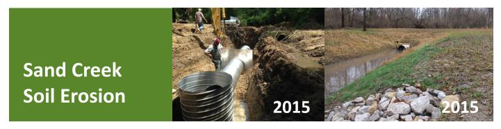
This drainage and erosion control project along a trail at Sand Creek Conservation Area was completed in 2015. It improves water quality, prevents soil erosion, and dangerous trail conditions by slowing the flow of water. As a result, less sediment washes into Lake Decatur, keeping our drinking water cleaner for wildlife and area residents.
